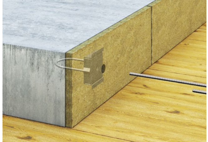
2. Remove shuttering and nails, apply max. 100 kg/m 3 mineral wool filler material.
