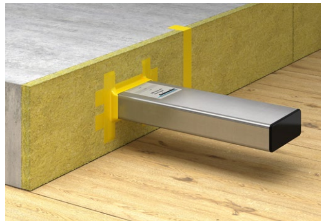
4. Mask the dowel and filler material joints.
